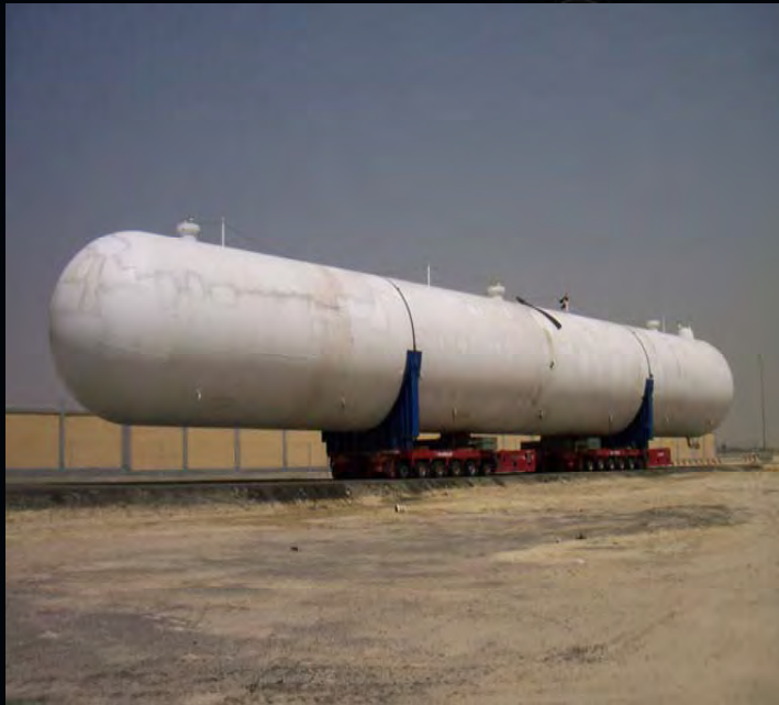
450 Ton Gas Bullet unit being transported to Site from Shuaiba-Kuwait
