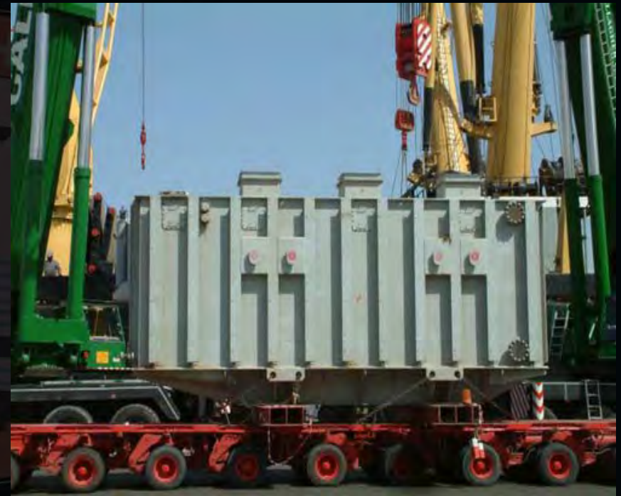
180 Ton transformer - tandem lift operation with 2 x 400 tons shore cranes to load onto the lower deck of vessel to Antwerp
